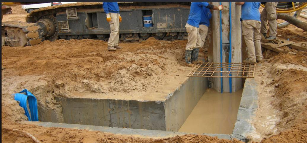
Stop-ends are easily placed to the ground and coupled together through special steel bars. They are made of sheet metal welded and internal pipes reinforcing the structure increasing its strength and toughness to prevent it from any damage. It is easy to connect or disconnect.
