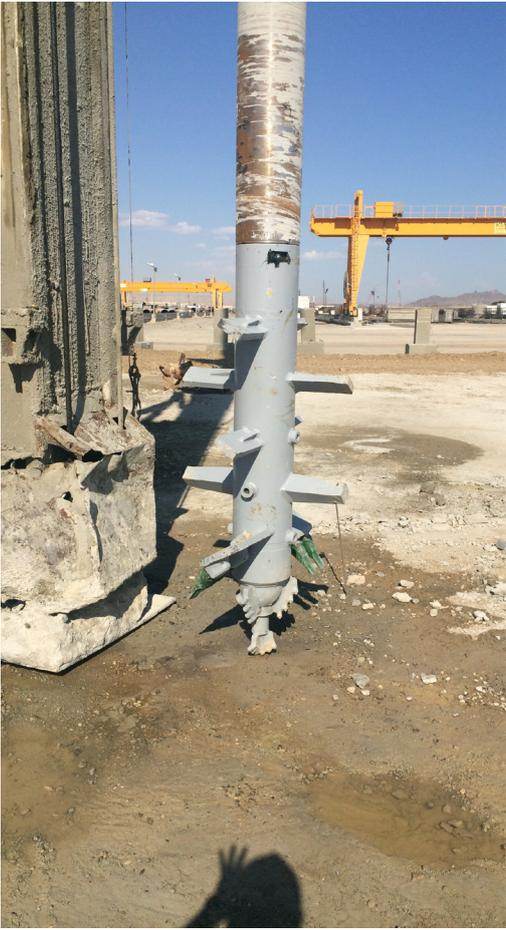
DSM method is an in-situ soil mixing technology that mixes existing soil with cementitious materials.
