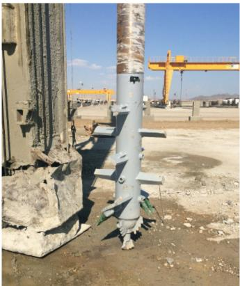
DSM method is an in-situ soil mixing technology that mixes existing soil with cementitious materials. DSM is effective for liquefaction mitigation of seismically sensitive soil layers, foundation improvement under future structures and in-situ stabilization of contaminated soils for environmental remediation among other uses.
