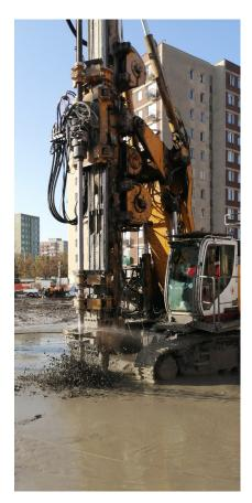
Z Makina has developed a jet grouting system with the single stroke columns to depths of 36 m capacity. It was designed which can be mounted on the piling rig used for jet grouting come in a range of different sizes; large ones, making it a perfect technique for improving the foundation of an existing structure.
