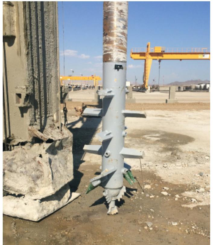
DSM method is an in-situ soil mixing technology that mixes existing soil with cementitious materials. DSM is effective for liquefaction mitigation of seismically sensitive soil layers, foundation improvement under future structures and in-situ stabilization of contaminated soils for environmental remediation among other uses.
